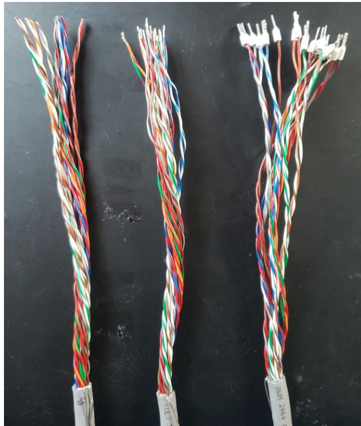
Ferrule-to-ferrule cables with cut (left), stripped (center), and terminated (right) ends
